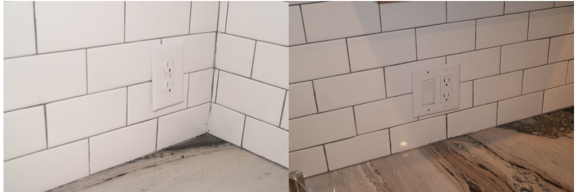
Receptacles in the kitchen were not secure to the wall.
