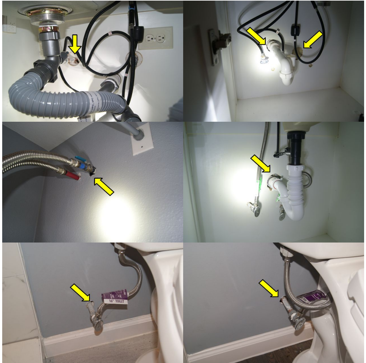
Walls under sinks were damaged and pipe penetrations did not have flanges to cover the gaps around the pipes.
